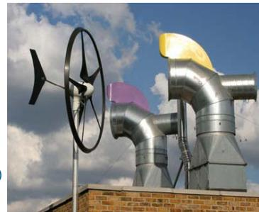
Micro Wind Turbine and cowling for passive ventilation system. Bedzed, London, UK
